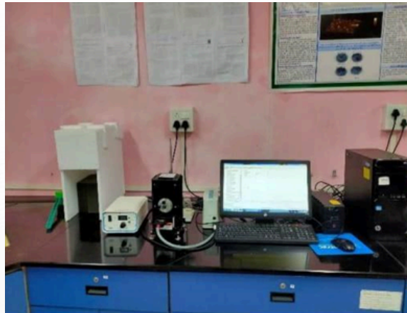
Solar PV Device System
